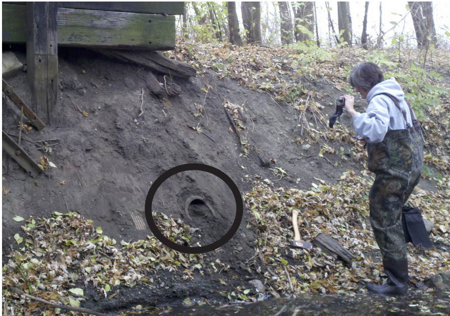
Toxic pipe discharge on bank of Boneyard Creek
